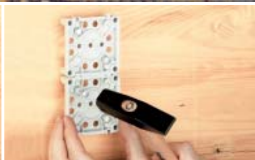
◀ + ◀◀ For the installation of back mounted boxes, the blank base is first fixed to the working formwork.
