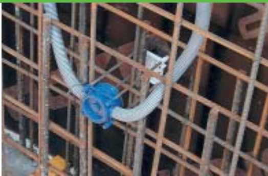
◀ Vertical installation in site cast concrete structures.
