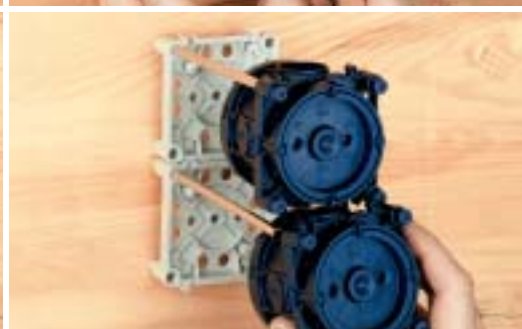
◀◀◀◀ Finally the boxes are pushed on, reversed.
